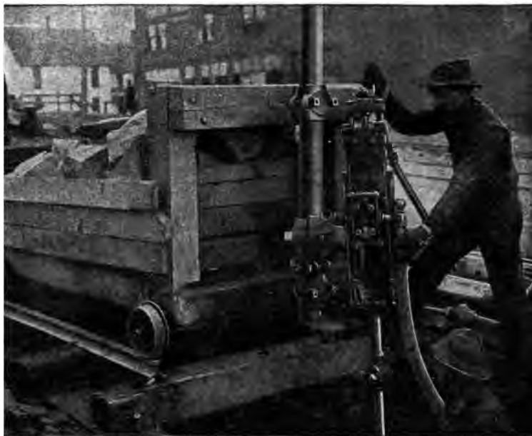
Fig. 166. Drill Carriage for Trench Work.
